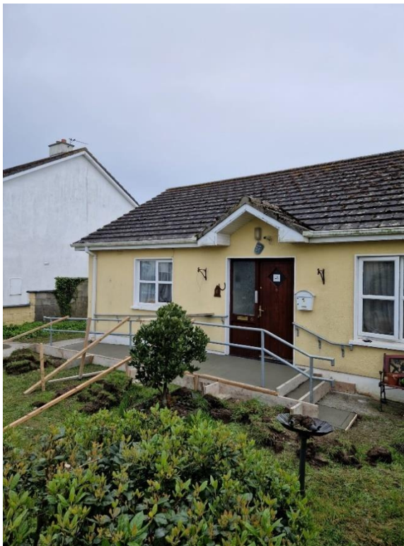
SAMPLE DPG WORKS TO EXISTING COUNCIL HOUSING
