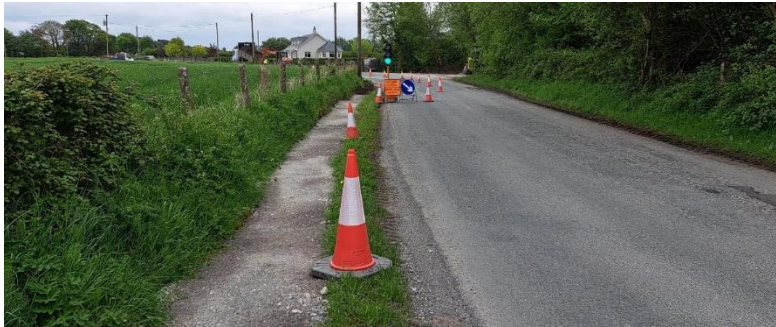
After – Works ongoing
