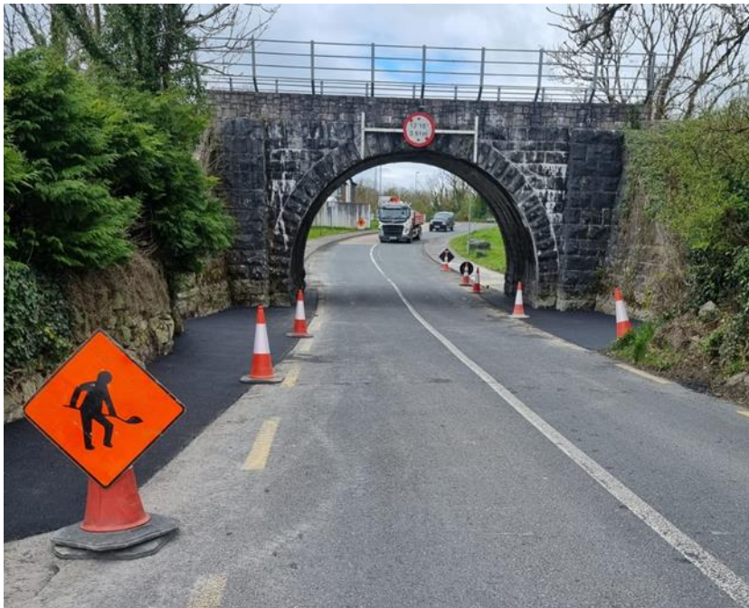
PEDESTRIAN IMPROVEMENT WORKS COMMENCED AT BRIDGE UNDERPASS, CRAUGHWELL VILLAGE
