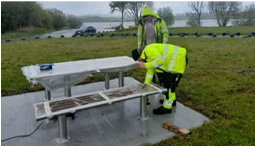
INSTALLATION OF NEW PICNIC BENCH AT THE LONG POINT, LOUGHREA
