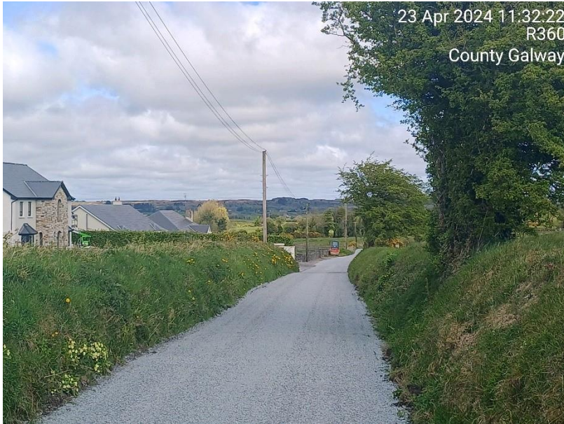
ROAD SURFACING AT L-22301 MEENLENA
