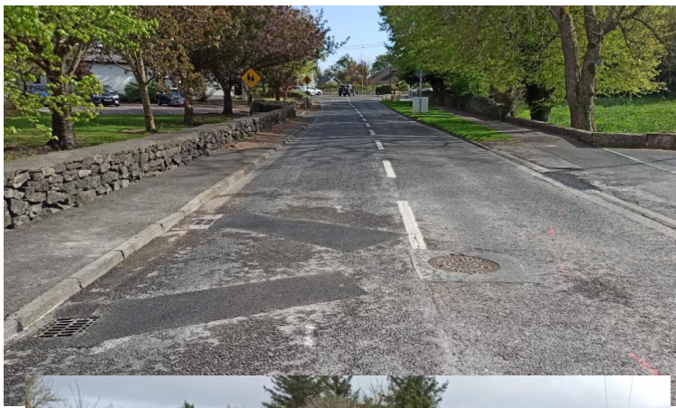
DRAINAGE REPAIRS ORANMORE
