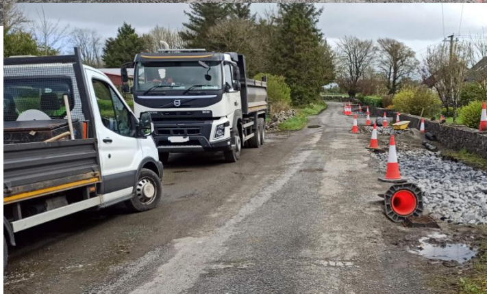
DRAINAGE WORKS CASTLE ELLEN
