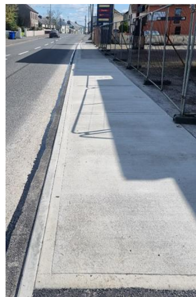
FOOTPATH IMPROVEMENT WORKS, CRAUGHWELL VILLAGE
